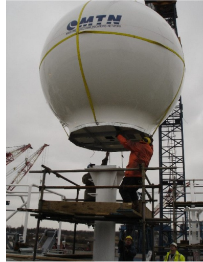
Satellite Dish Being Installed
