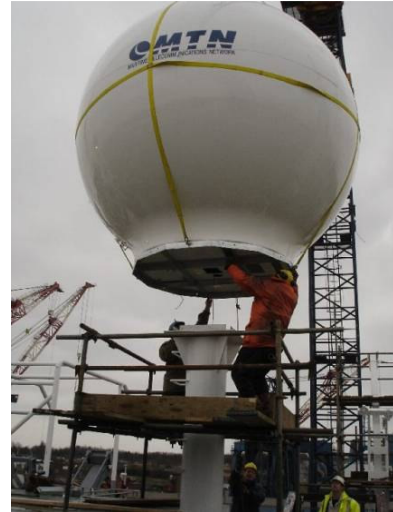
Satellite Dish Being Installed
